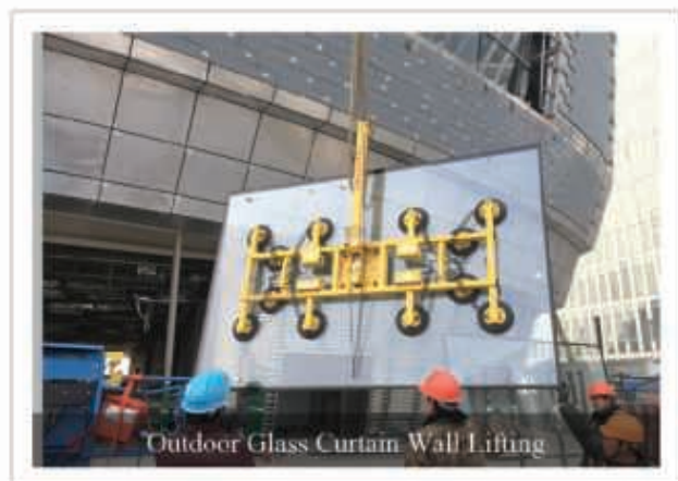
DC-Vacuum Lifter (12 Suckers) FS-SFX1200-12S (1200KG)
