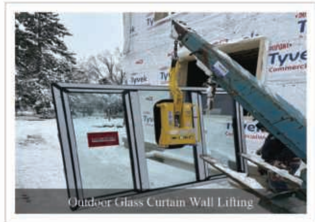
DC-Vacuum Lifter (Single Sucker) FS-SFXi500-IS (500KG)
